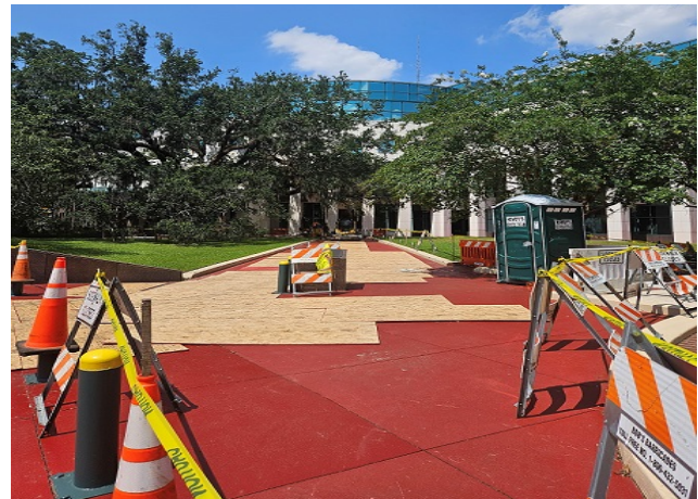
Building Infrastructure and Improvements - Courthouse Plumbing Repair
