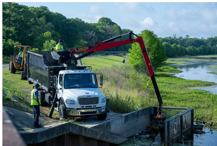
Stormwater Pond Repairs
