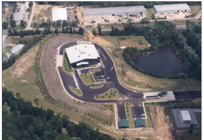
Leon County Transfer Station
