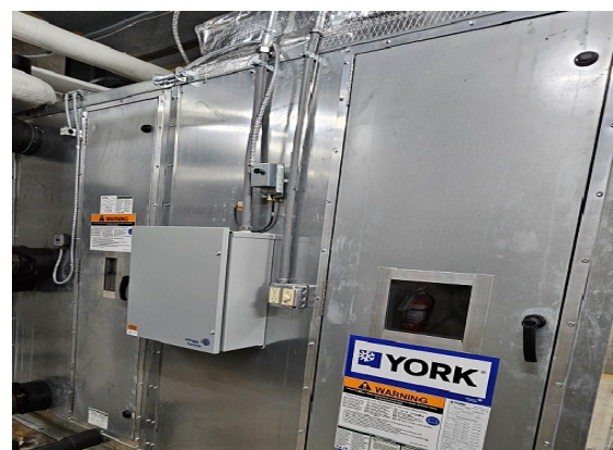
Building Mechanical Repairs and Improvements - Air Handler
