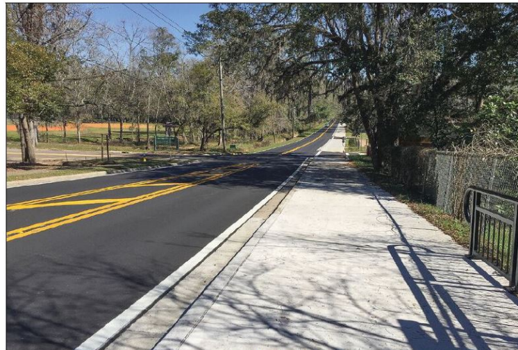
Local Road Resurfacing
