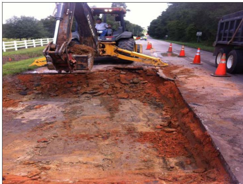
Asphalt Road Maintenance
